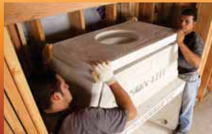
4. Finishing with the dome top
