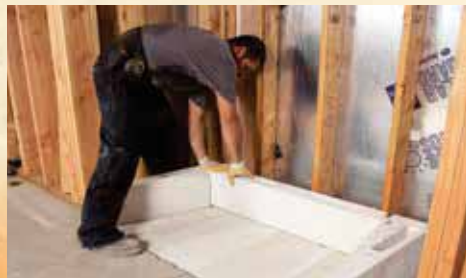
1. Installing base and first course
